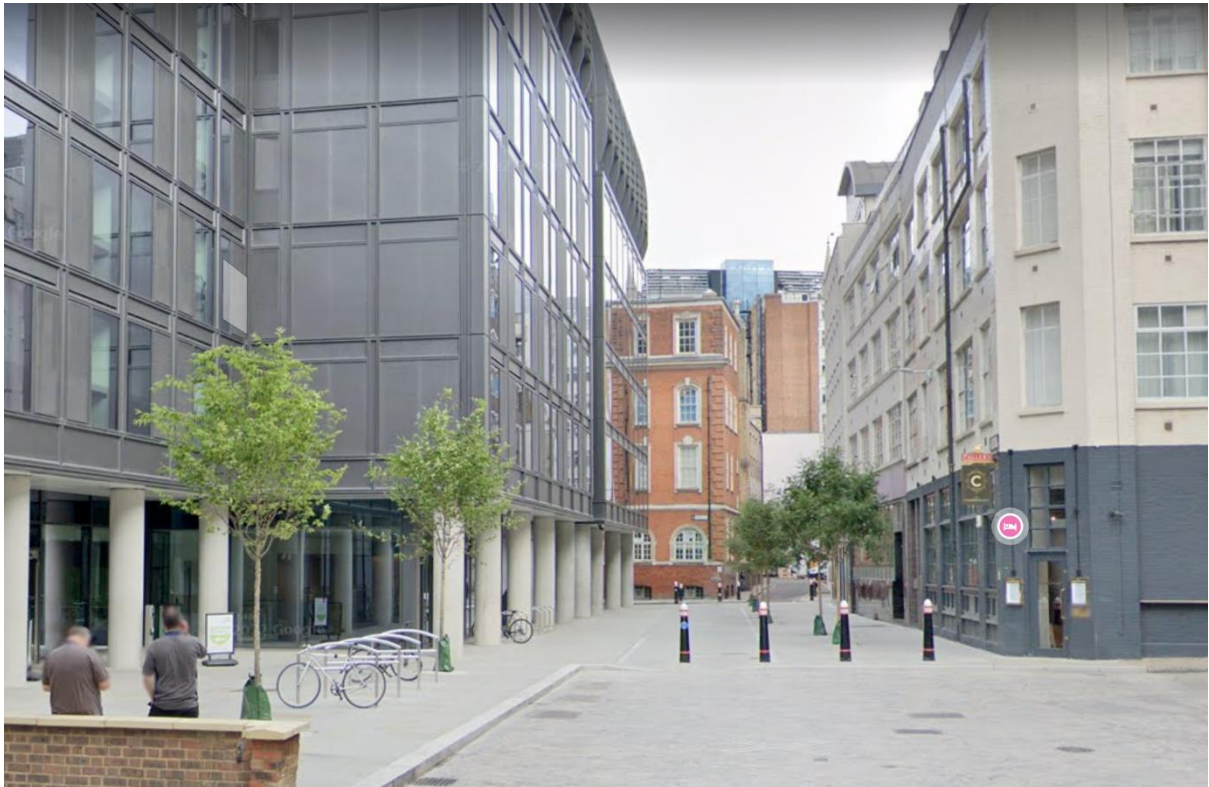
Looking north after scheme completion
